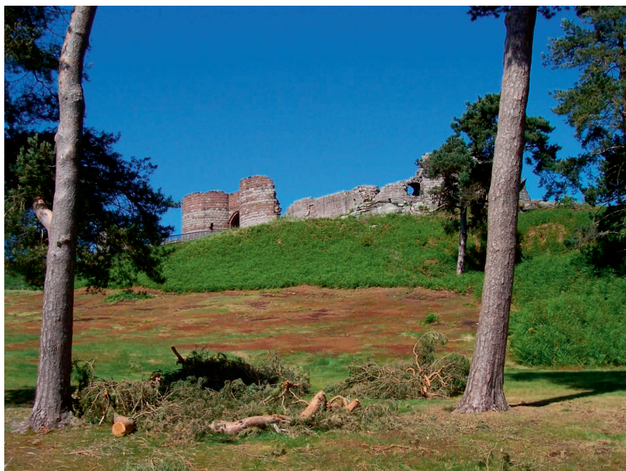
Plate 9: Taken from the outer ward, looking towards the inner, this photograph conveys both the unusually large extent of the outer ward and the way that it slopes, albeit more gently than the steep hillsides below, rising up to the inner ward at the highest point of the summit.
