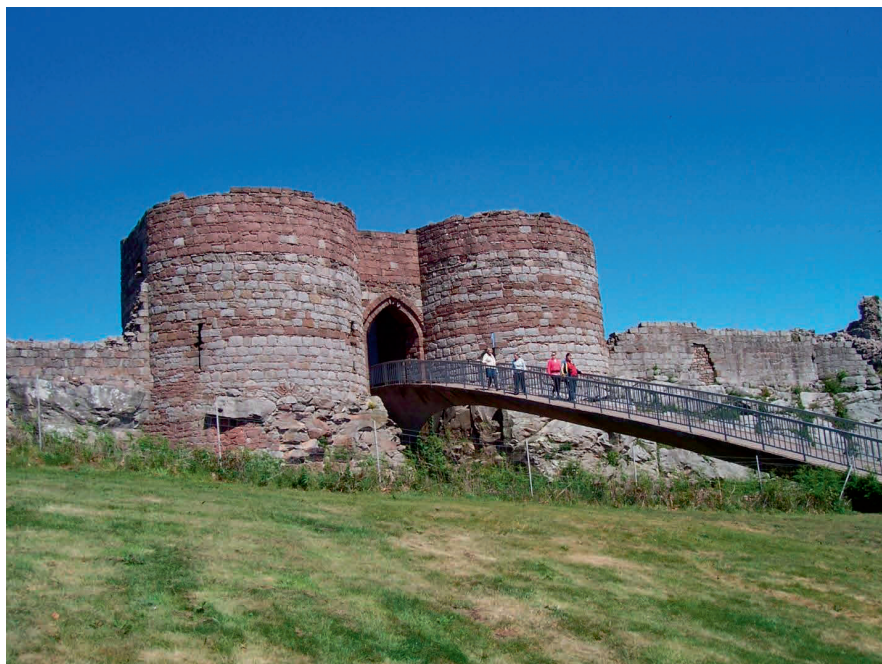
Plate 7: Looking north from the outer towards the inner ward, the twin-towered inner gatehouse, now accessed by a modern bridge, was constructed from regular courses of stone, much of it the distinctive red sandstone of Cheshire's sandstone ridge.
